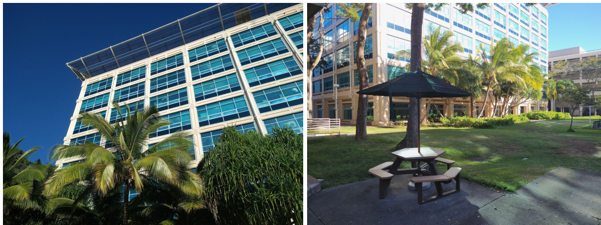
The Pacific Ocean Science and Technology Building, home of the Dept. of Earth Sciences
