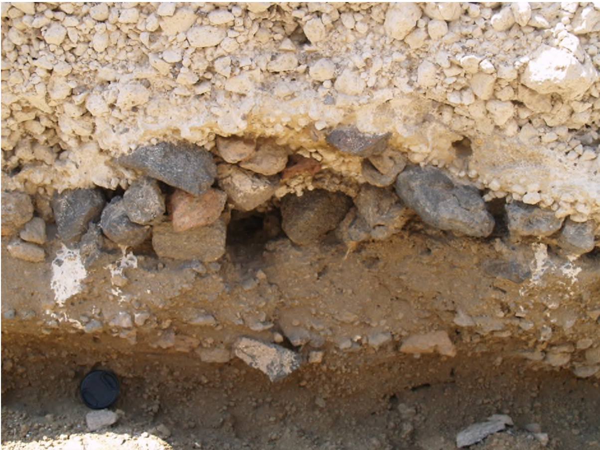
Figure 30 Pulse 2 and 3 deposits draping an old agricultural wall. Pulse 2 deposits are incorporated in the base of the Pulse 3 deposits. Picture taken from an exposure within the Akrotiri Quarry.
